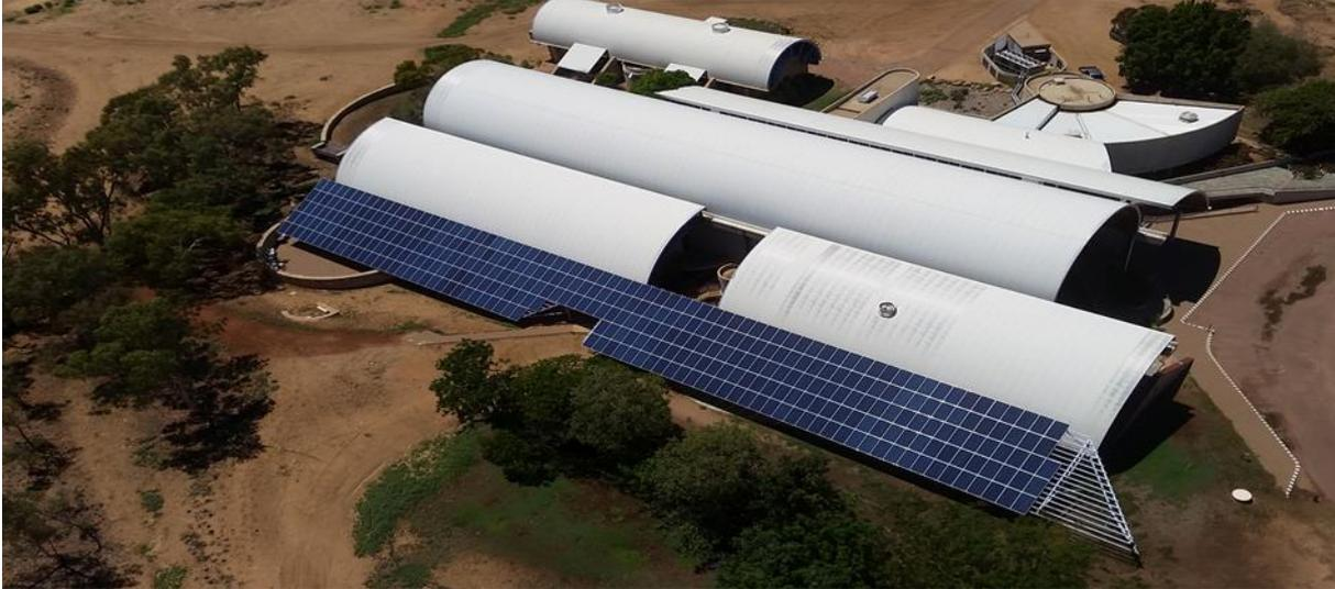
With temperatures reaching over 45 degrees the team installed over 350 panels over four weeks. Utilising the existing steel structure located on the north of the building
