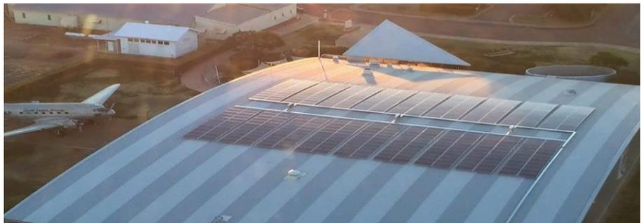
The installation was completed over three months and comprised of 318 Trina solar panels with 3 ABB inverters. Installed on the Museum roof utilising Clenergy rail, the installation can be seen to great advantage from above.
